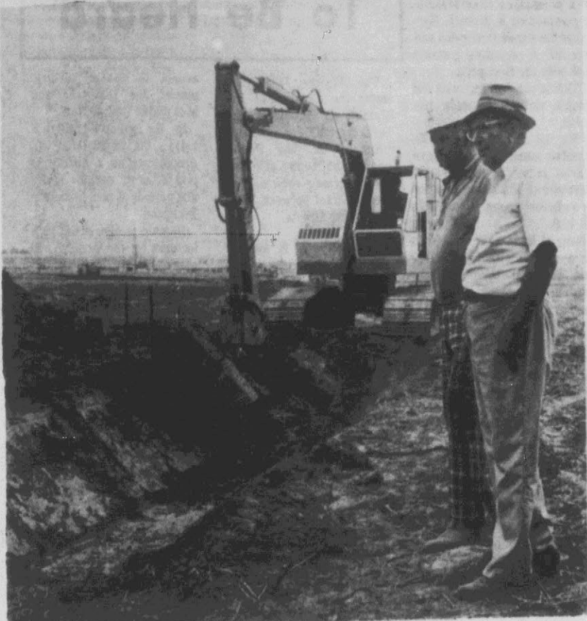
VISIT CONSTRUCTION SITE — Jim McFarlane, project supervisor, left and D. R. Hoke, grading contractor, visit the construction site of a storm water retention pond at the new Greenville Square Mall.
