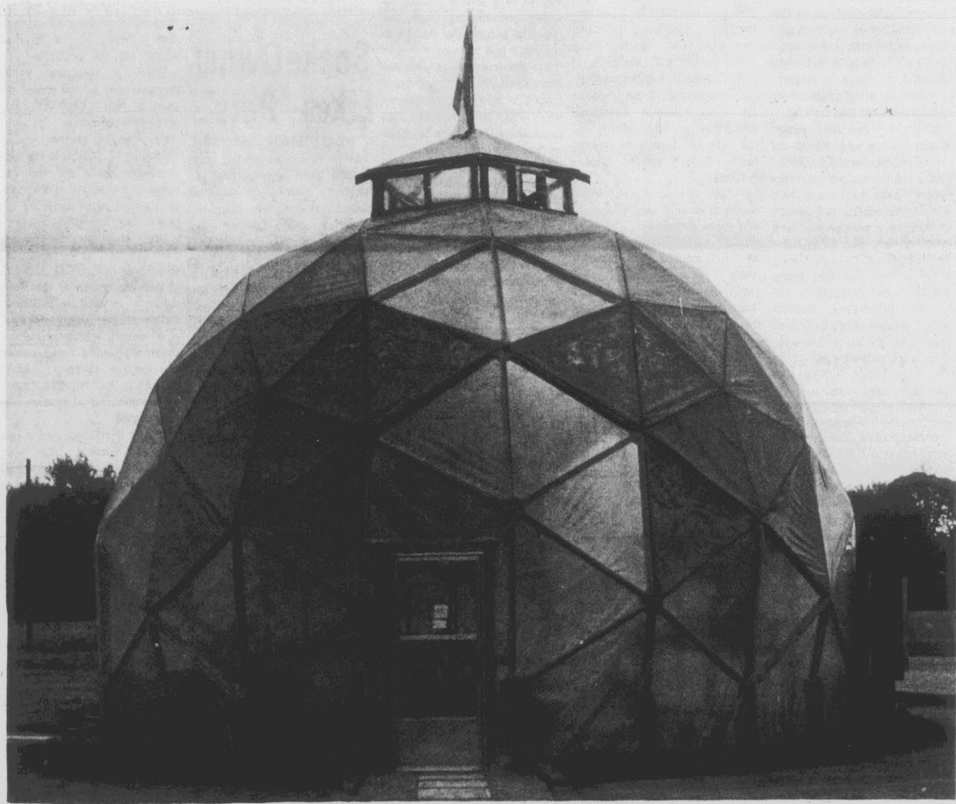
THE COMPLETED DOME . . . is covered with polyethylene plastic and used for a plant display building at Plant And See Nursery.
