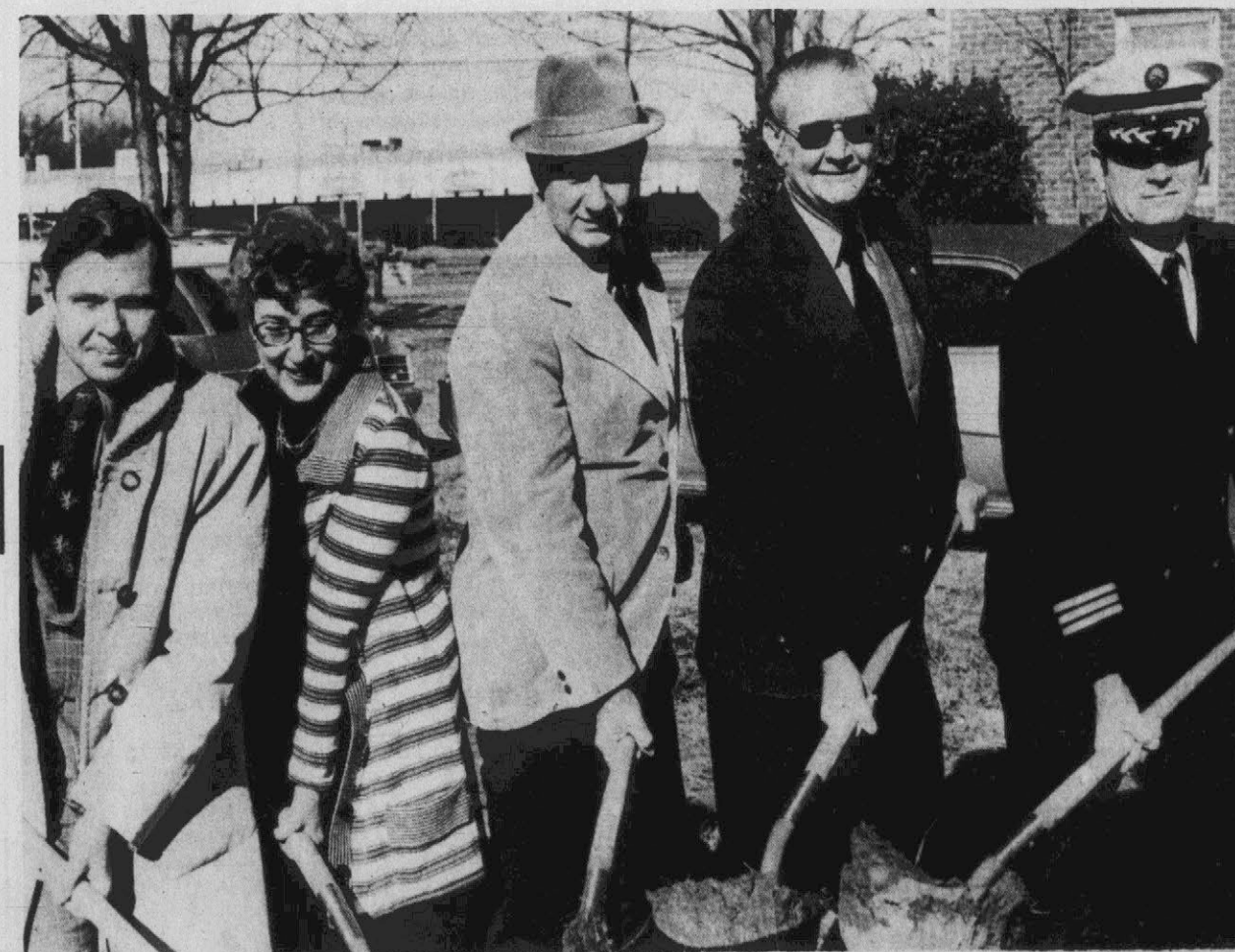
NEW STATION SITE—Taking part in groundbreaking activities Friday at the Memorial Drive site selected for the city's new fire station were (L-R) City Manager Jim Caldwell, City Council
